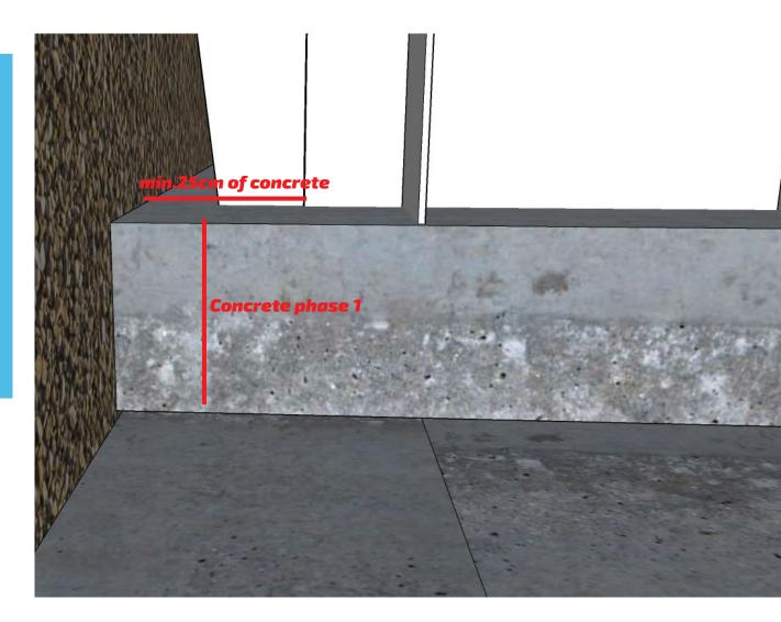
When concreting, it is necessary to pay attention to the pipes around the pool, concrete and other objects must not hit/tear off glued joints. (We recommend to carefully sprinkle the piping at first). During concreting, we recommend to check all joints around the pool and in the tech box.
